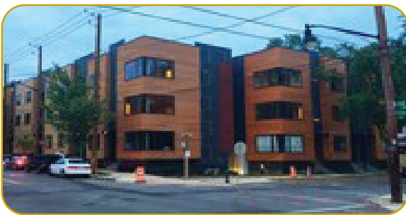
Example of stacked flats. This type of housing would be most appropriate on corridors in Berkley.
